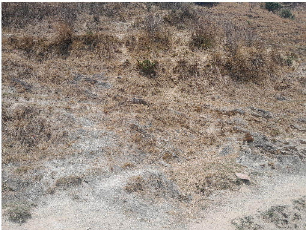
Highly weathered and fractured bedrock exposed in Khola Dhab.
