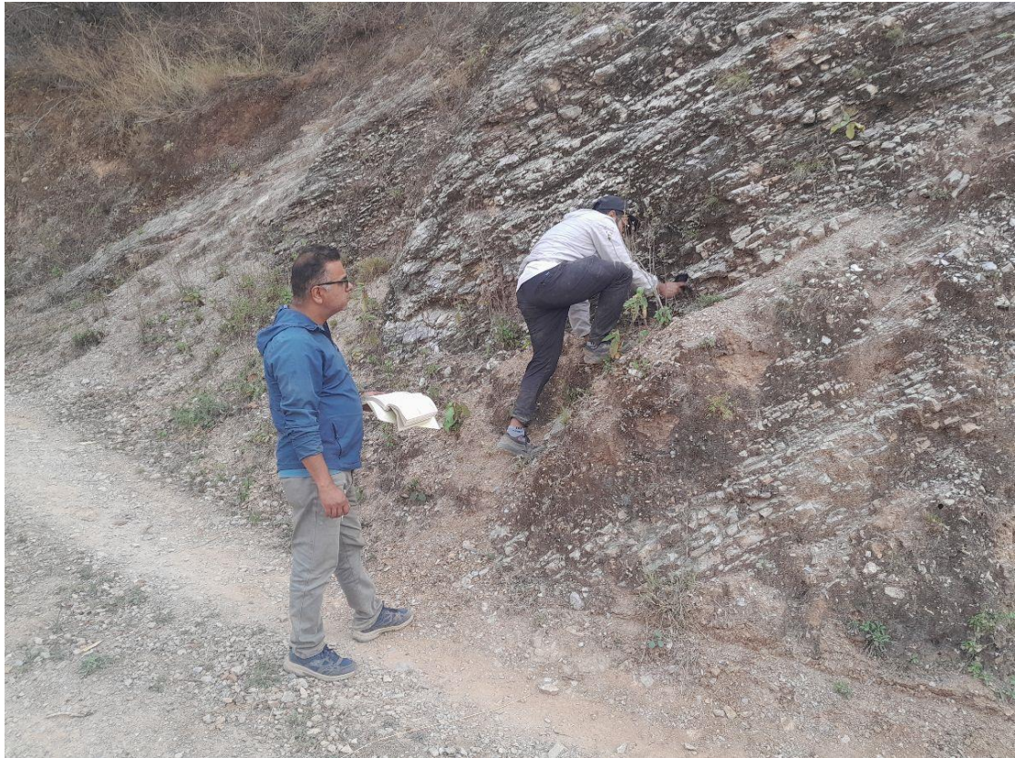
Bedrock exposed and data measurement in Lek Kurile landslide.
