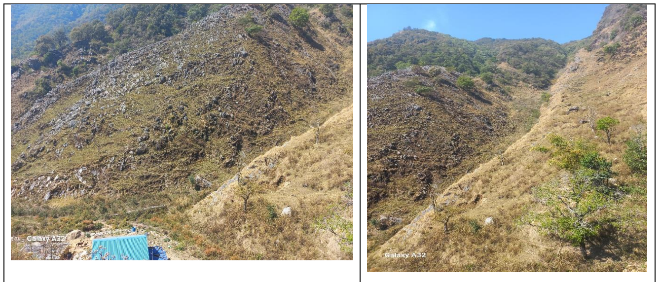
Figure 24: Photographs indicates the view of debris flow gully and risk zone of the Bhitrikhola landslide
