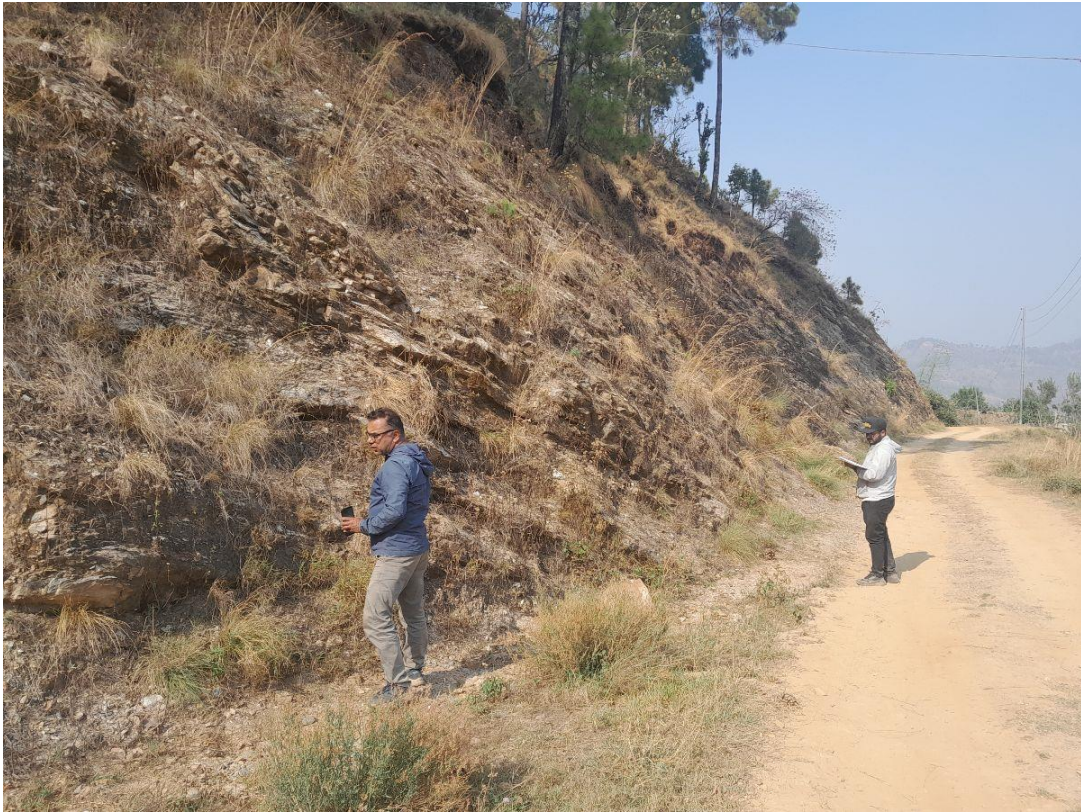
Bedrock exposed in Hile landslide in the road cut section.
