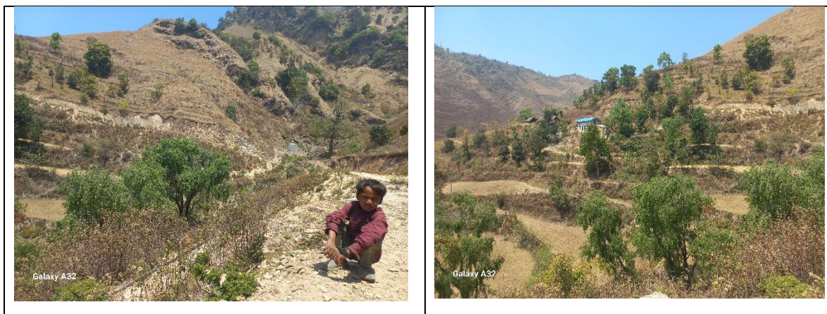
Figure 115: Photographs of instability area of Khola Dhab landslide zone
