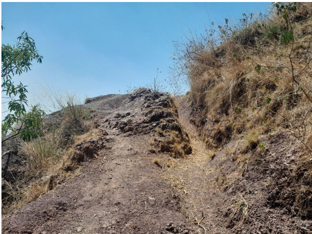
Highly weathered purple shale observed in the top portion of Lekh Malarani.
